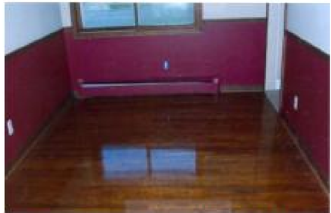
Interior Room Clean of Debris
