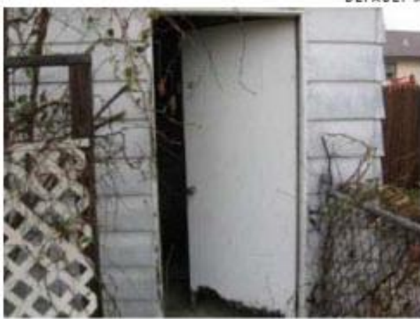
Security Door Before
