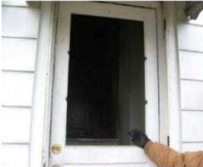
Door Boarding Before
