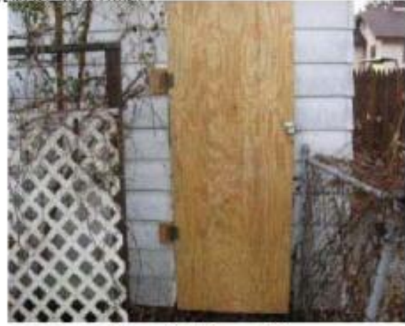
Security Door After
