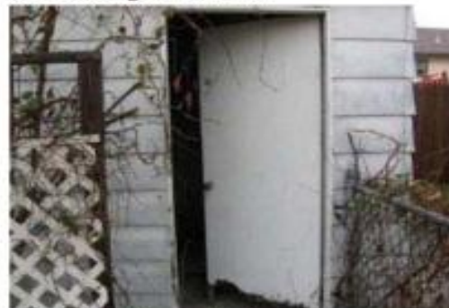
Bid to install security doors
