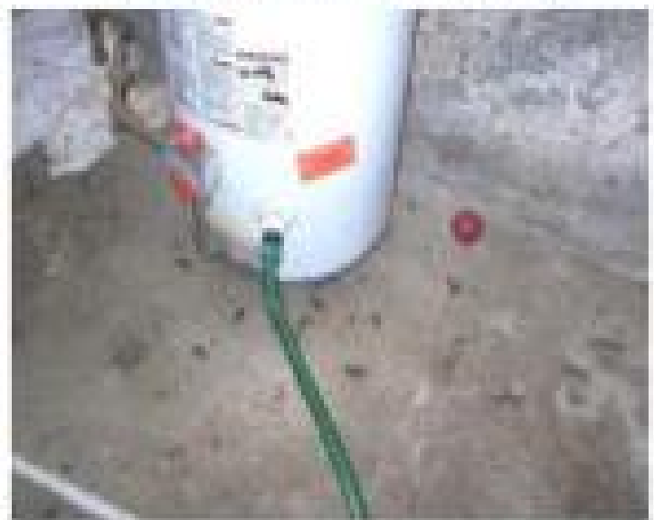
Winterization - Water Heater After
