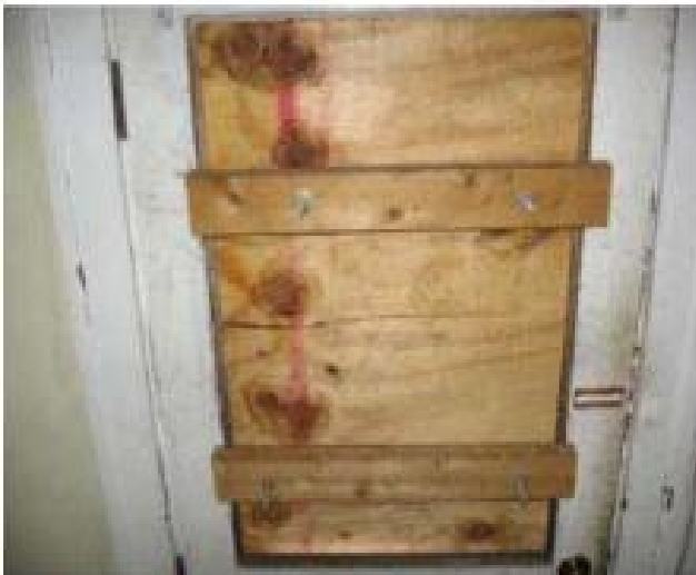
Door Boarding Interior After
